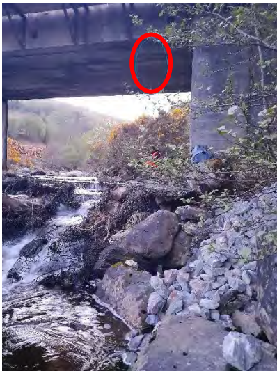
Photograph 21: Location of pipistrelle bat emergences at Kilfinnan Bridge.
