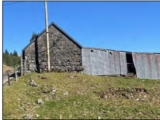
Photograph 16: Barn at North Laggan
