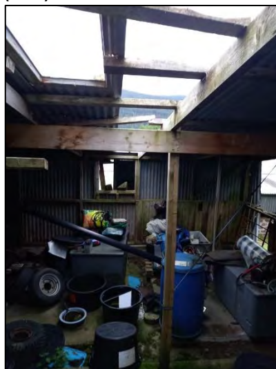
Photograph 24: Interior of metal lean-to on south aspect of the Barn.
