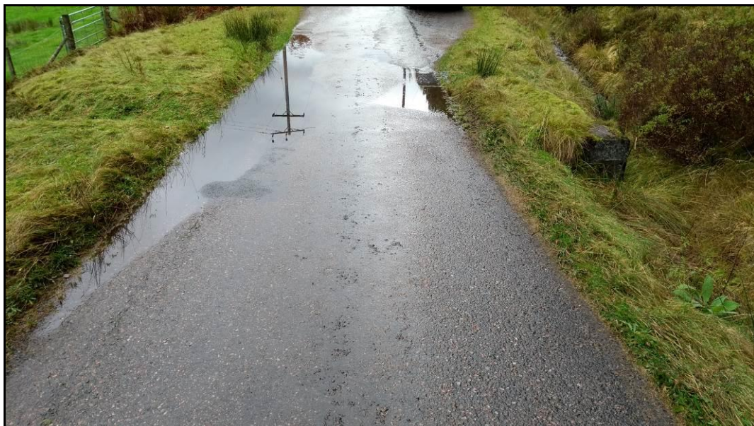
Plate 14.11: Surface Water Ponding on Public Road along the West of Loch Lochy
