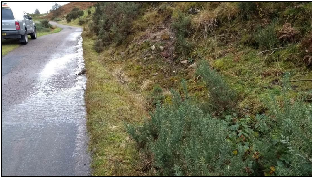
Plate 14.12: Road Drainage Ditch Overflow on Public Road Along the West of Loch Lochy
