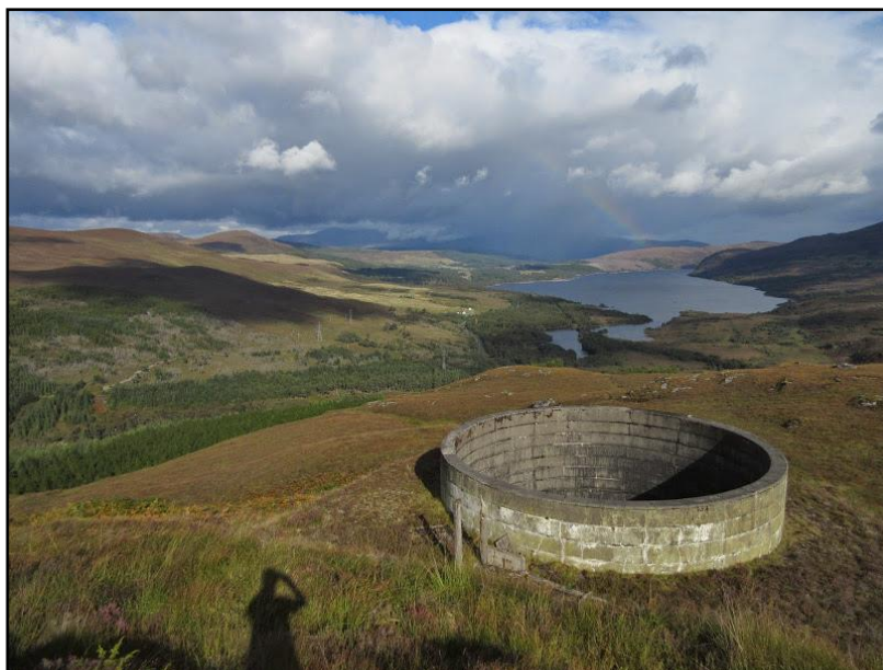
Plate 3.4: Example of a Surge Shaft
